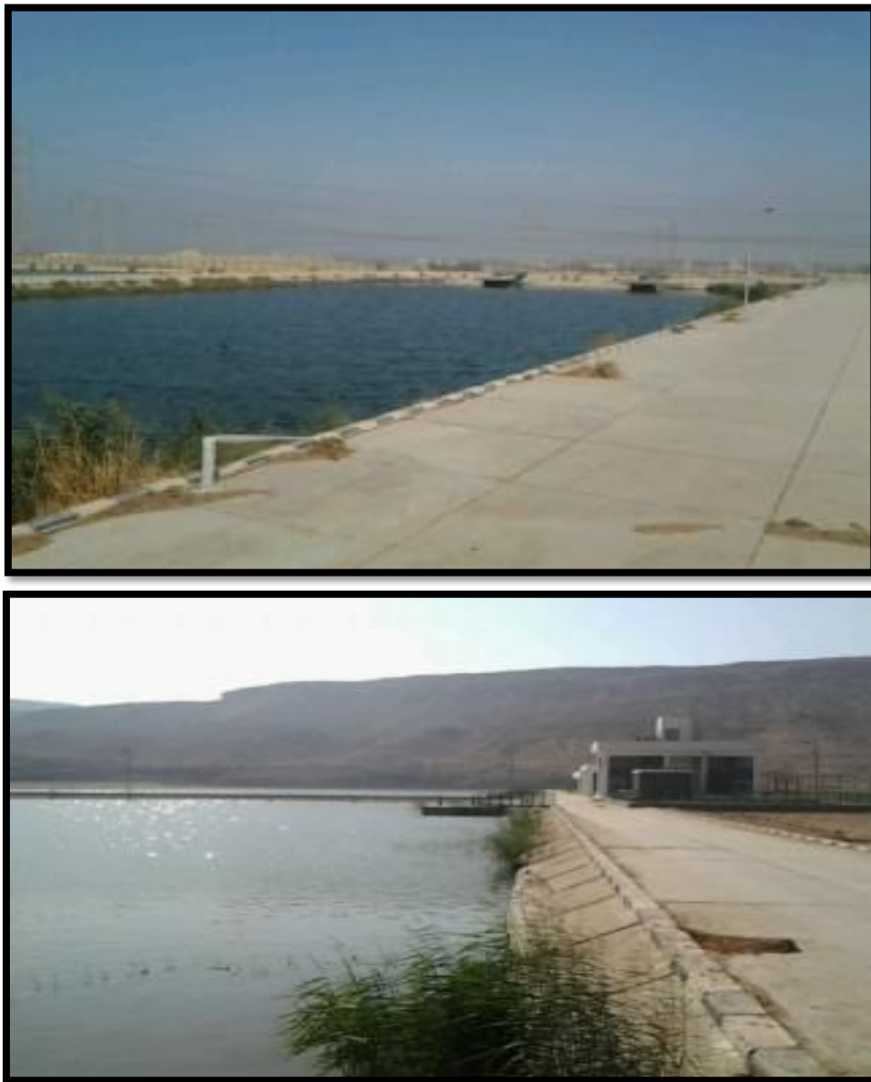
Fig. 1. Elzaraby Waste stabilization ponds.
